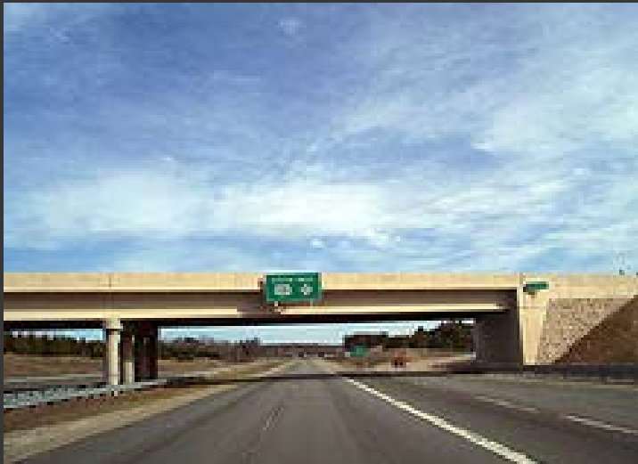
M-55 bridge over US-131 as it joins the Cadillac bypass
