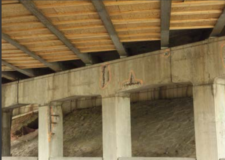
Plywood Under I-375 Bridge
