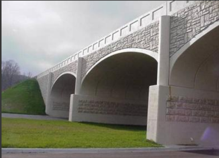
US-31 bridge in Beulah
