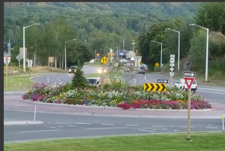
US-41 roundabout in Marquette
